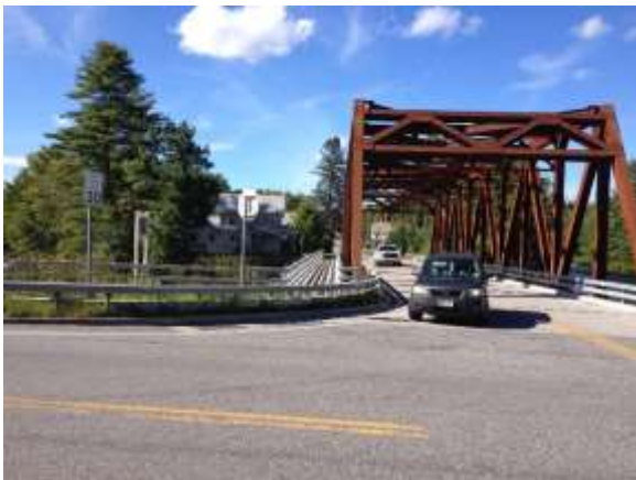
Bridge at Milton St. View north
