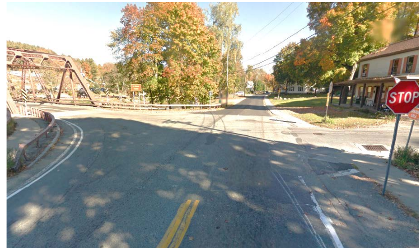
Poor striping, no stop lines, lack of crosswalks, wide turning radii, and an awkward stopping configuration make for seemingly unsafe intersection (courtesy of Google Street View)
