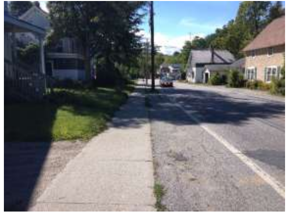
East of South St. View west
