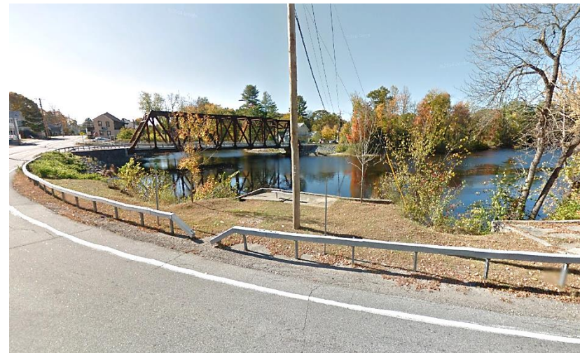
With no sidewalks and only small gap in the guiderail, the small pocket park located opposite the Alden Avenue intersection has limited accessibility (courtesy of Google Street View)
