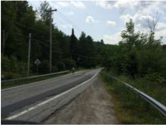
At pull off near substation View west
