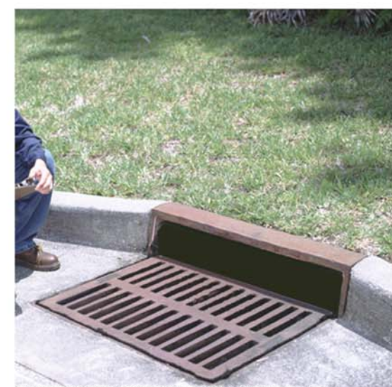
INTEGRATED CATCH BASIN / CURB INLET
