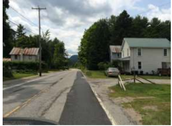
East of substation View west
