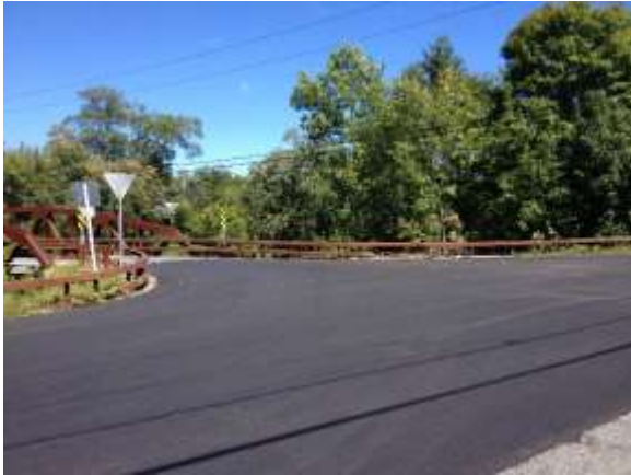
Judd Bridge View northeast
