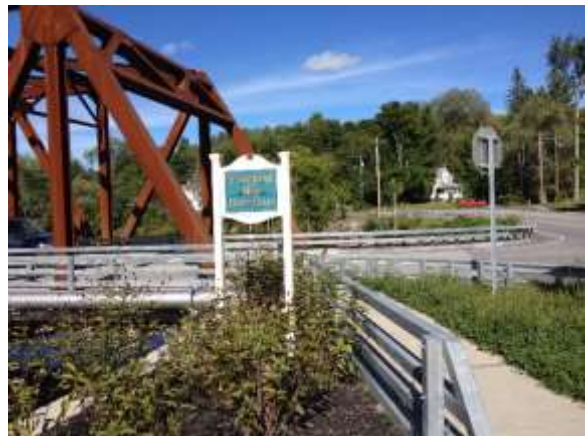
Bridge at Milton St. View east
