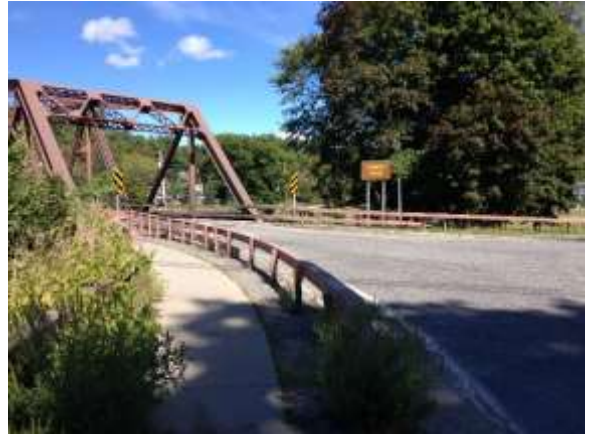
Bridge at Richards Ave. View northeast
